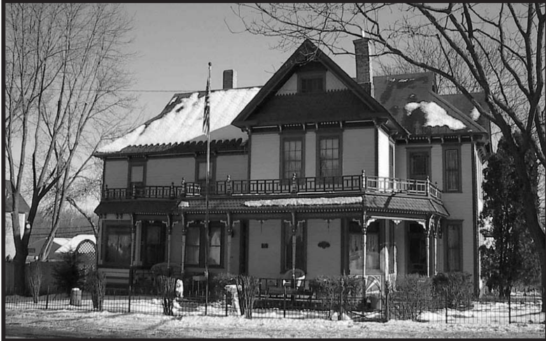
The east (left) side of the house was built in 1856-57 and was probably the Levi H. Griffin family residence from 1857-1876. Griffin's brother-in-law, Joshua P. Torrey and his family, lived in the west side of the building. In 1876 the Torreys came to own the entire building. By 1893 the John Hebeisen family had ownership and smoothly fit the entire structure(s) into an Eastlake Queen Anne Revival home. The house, often called the Gables, survives on Fourth Street East in the Carver Historic District and is listed on the National Register of Historic Places. Shown here in 2005. (JvW)
